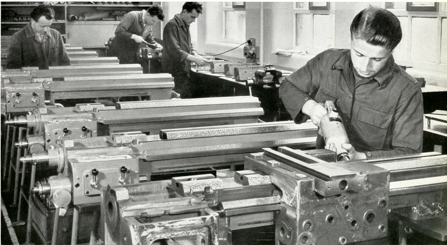
Assembling the bed and carriage
